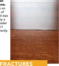
Small cracks can be filled. A board with cracks in its face doesn't always need to be replaced. The board shown here may be repaired with a touch-up kit.
