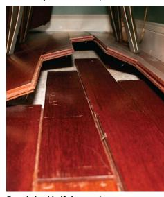
Boards buckle if they can't expand. When floorboards aren't acclimated or are exposed to lots of moisture, they can crush together and lift off the subfloor.
