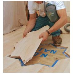
Cutting corners. A corner chisel squares off rounded corners left by the router bit.
