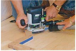
**Don't cut all at once.** Several shallow passes with the router cut through the flooring safely and easily. Above, a crew member holds a vacuum to keep dust and mess to a minimum. After the final cut, the waste is removed (photo right).
