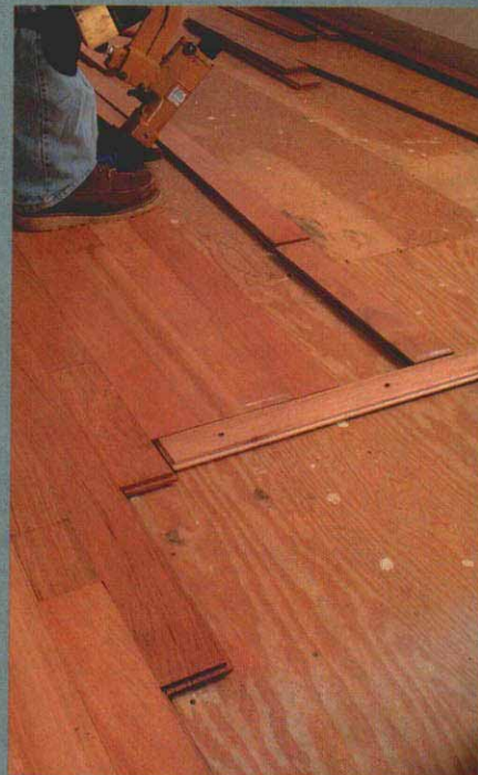
A temporary stop establishes the border's line. Screwed into the subfloor, scrap flooring provides a clean starting point for the flooring and a fast, straight line for one side of the floor's border.
