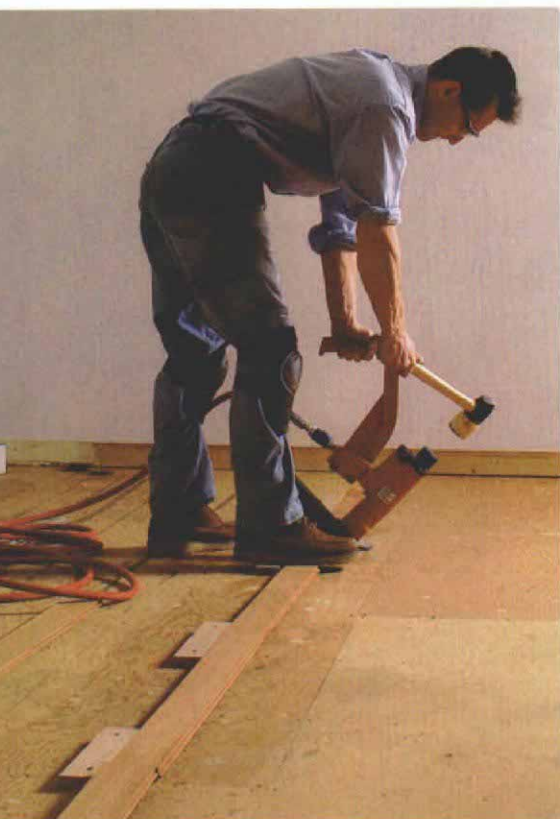
Reverse the flooring's direction with a slip tongue. Lengths of hardwood splines are glued and pinned into the groove of a center starter course. The flooring can then be nailed down in the opposite direction.
