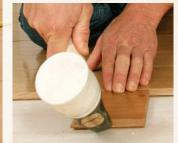
Use a bash block made of scrap flooring to knock stubborn boards into place. The matching profile ensures that you won't damage the delicate edges of the floorboards.
