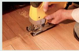
Drill holes near the edge of the damaged board and use a jigsaw to crosscut it.
