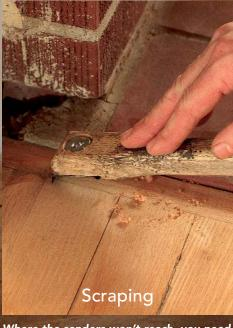
Where the sanders won't reach, you need to scrape. A sharp carbide blade works well, although it's hard work.
