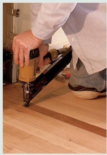
Hammer the old nails into the subfloor. Make sure the subfloor is absolutely clean with no high spots. Glue in the replacement with construction adhesive or a quick-drying epoxy. Because construction adhesive takes longer to cure, you'll need to weight down the replacement board overnight while the adhesive sets up.
