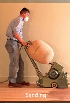
Going from coarse grit to fine removes the existing finish and leaves the floor ready for a new one. Drum sanders and edgers can be rented.
