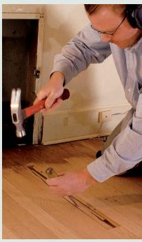
Use a chisel to remove the pieces of the old board. Always remove the pieces working away from the good floorboards.
