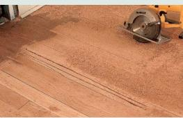
With a circular saw, make two cuts down the length of the board.
