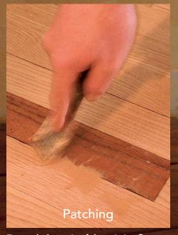
To match the grain of the existing floor, the author uses a replacement board from a closet where a new wood patch won't be noticed. After replacing damaged floorboards, he fills nail holes and cracks to prepare for sanding.
